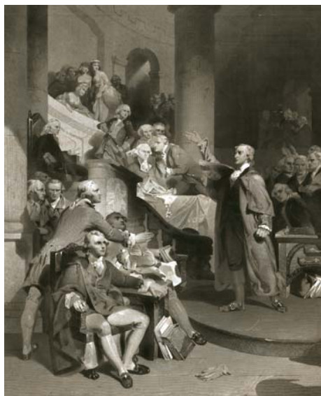
◀ Virginia gentry in the House of Burgesses
